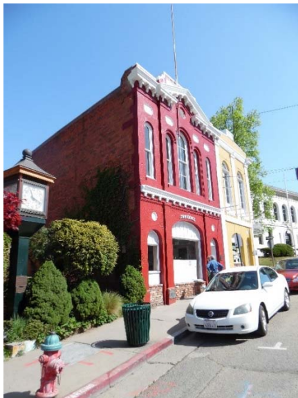
Figure 158 - Old City Hall Building
