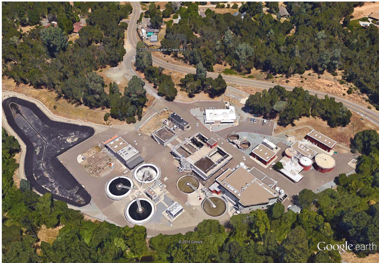
Figure 23 - Aerial View of Wastewater Treatment Plant
